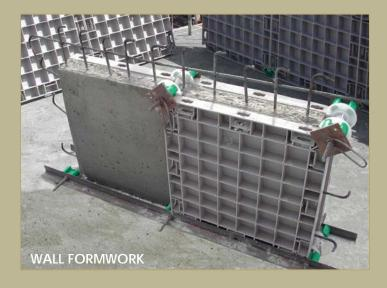
The formwork process designed and developed by DC INTERNATIONAL is modular and consists of several components of varied sizes, making it possible to set up concrete buildings from one to four stories of almost any dimensions.
